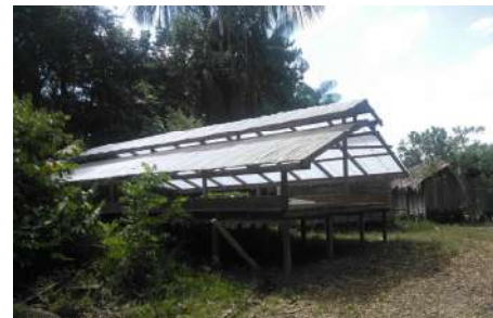
Fig.20 A. Portaccio, stove effect warehouse for the nuts' drying
